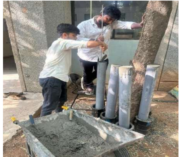
Fig 5.2 Casting of Column
