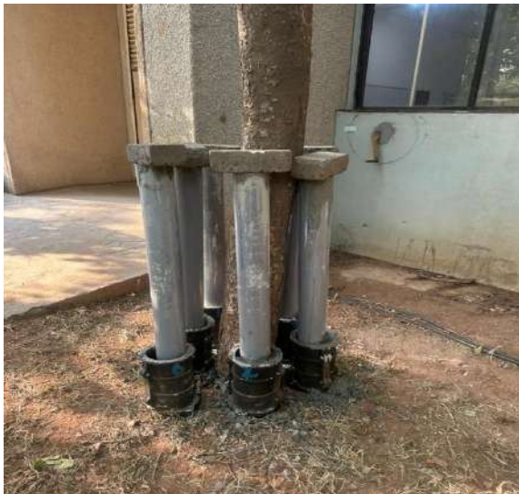
Fig 5.3 Column Casting process
