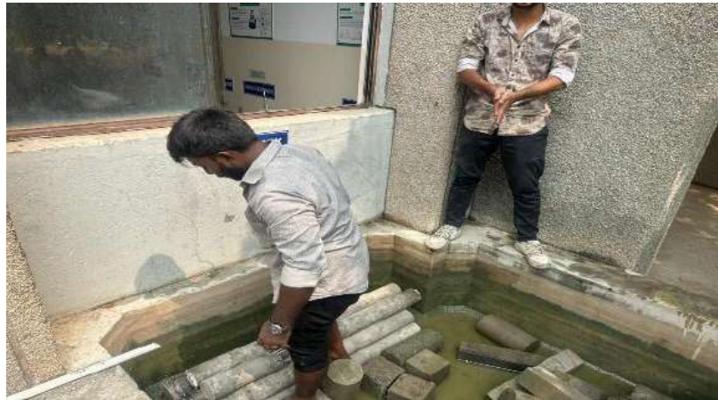
Fig 5.5 Curing of Column
